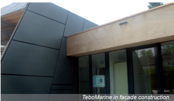
TeboMarine in facade construction
